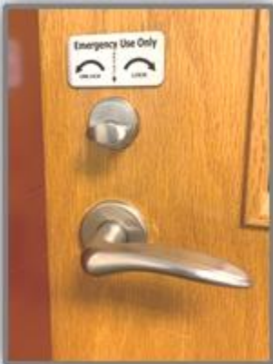
General Classroom Emergency door lock
